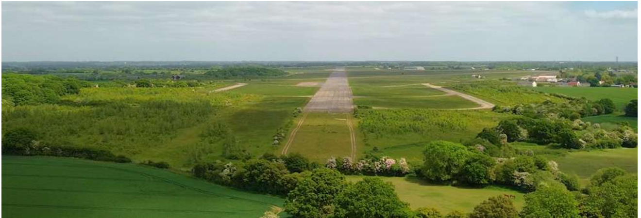
Figure 56b: LCA B9 Airbase 246 Looking down the runway showing its reintegration into the landscape.
