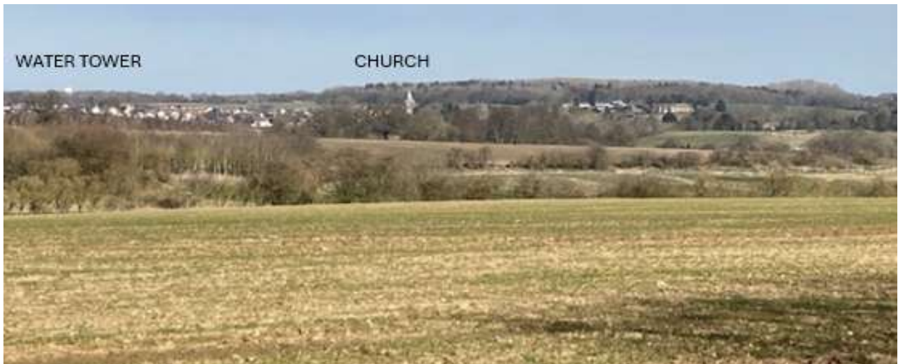
Figure 57b: LCA A5 Pant Valley 249 View from Hulls Lane across the Pant Valley towards Wethersfield with the church in the centre set against the rising profile of Poor Wood and the airbase water tower on the left horizon.
